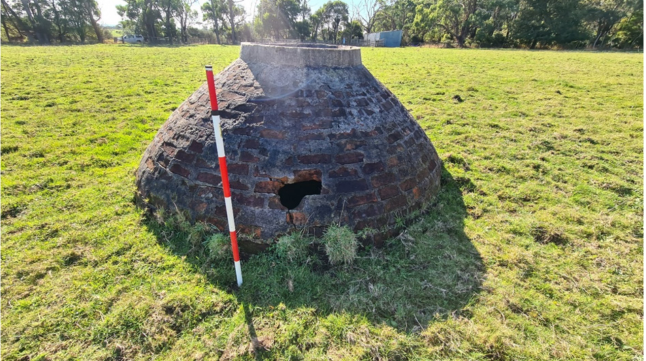
Plate 4-05 Brick cistern, located in Buffalo (view north-east)
