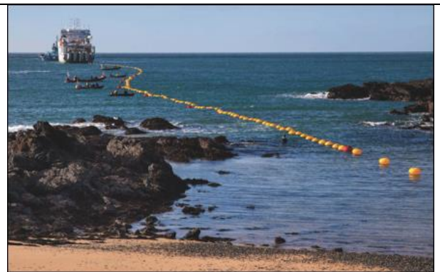
(b) Small boat fleet manoeuvring floated cable
