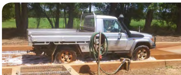
An automatic vehicle wash down bay provides protection against soil borne diseases.
