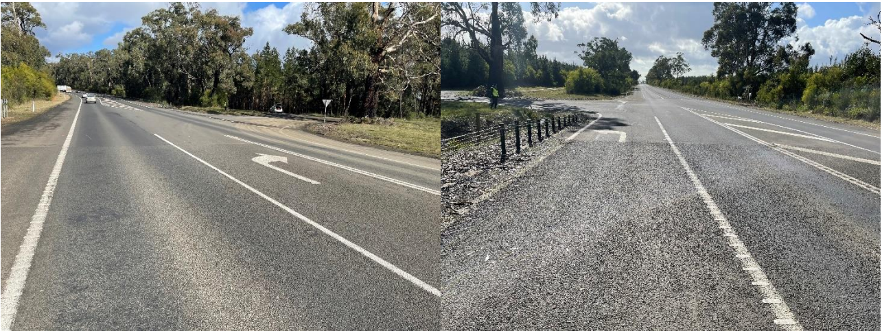
Figure 7.10: Photos taken at the Smiths Road / Strzelecki Highway Intersection on 23/08/2022
