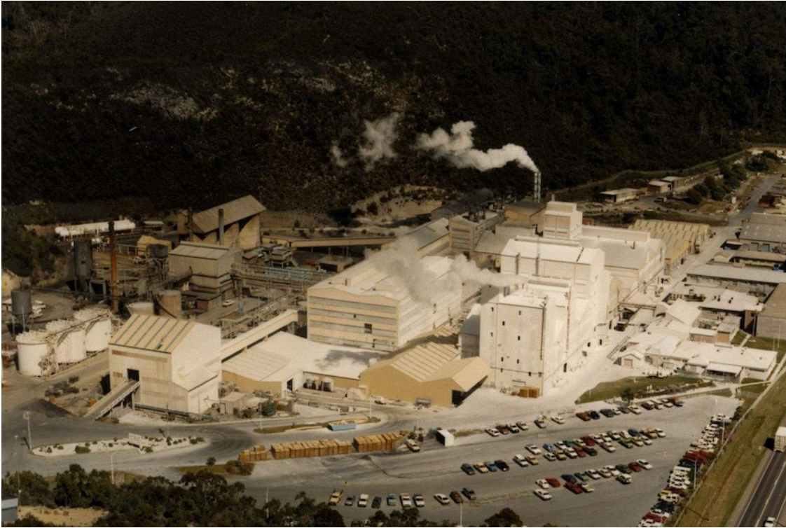
Figure 6-1 Photograph of the former Tioxide Australia manufacturing facility (ABC Radio Hobart, 2022)
