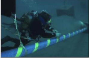
(a) Bellmouth being attached to HDD duct
