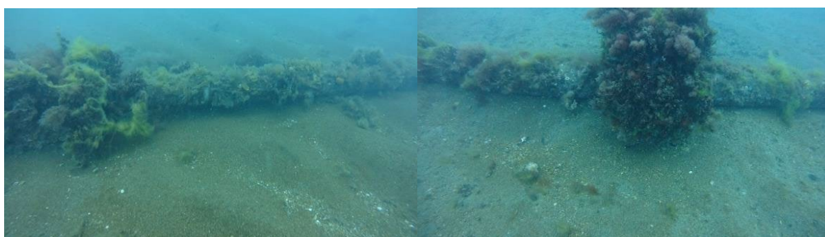
Figure 5-18. Disused Tioxide pipeline at Blythe River, January 2019 Left: Site W09, (12-13 m depth), Right: W08 (15-16 m depth)
